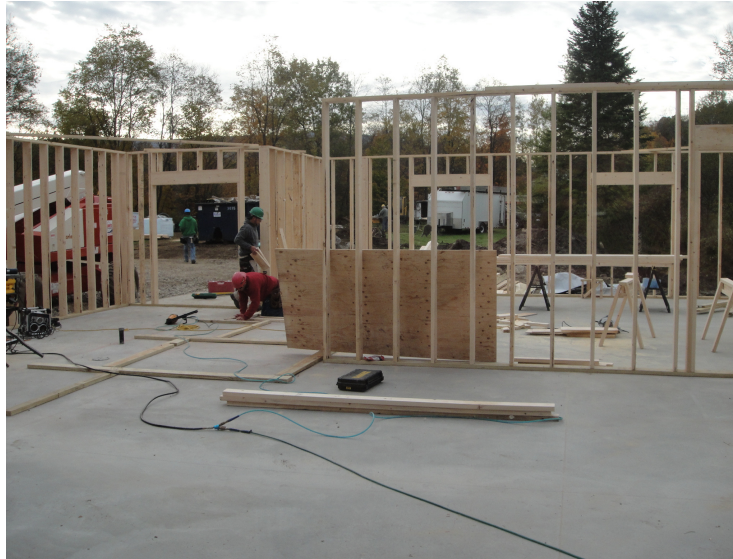
Framing the 3 rd and 4 th grade classrooms, September 2011
